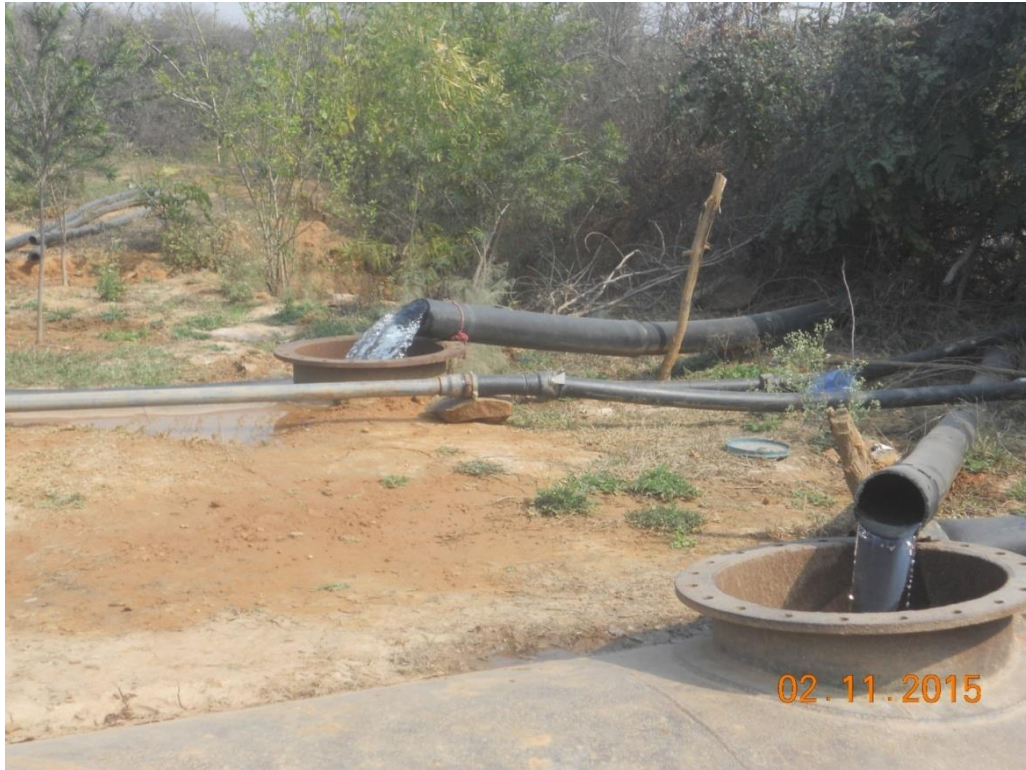
Underground tanks for the storage and distribution of irrigation water
