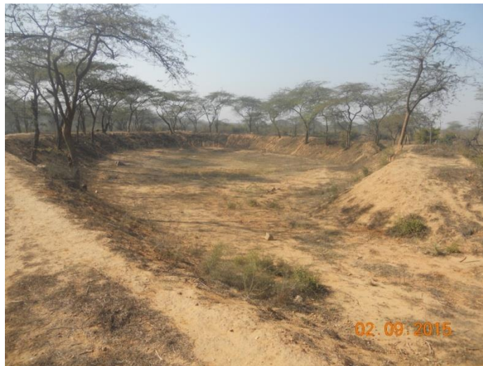
SMC Work (Inlet of water pond)
